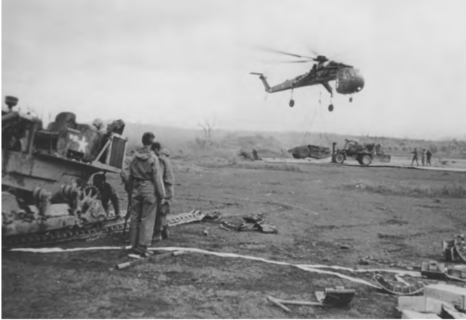
At Khe Sanh Airfield, a CH-54 Flying Crane drops off sectionalized engineer equipment.
